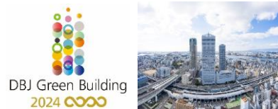
Art Hotel Osaka Bay Tower & Solaniwa Onsen 1
