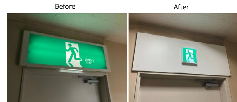
(LED conversion work of emergency exit signs at Hotel MyStays Sapporo Aspen)
