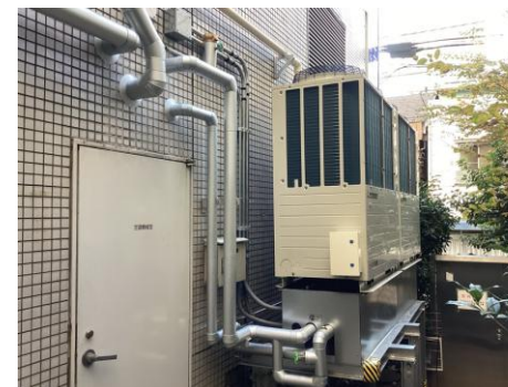
(Hotel Mystays Ueno East, highly efficient heat pump hot water systems)
