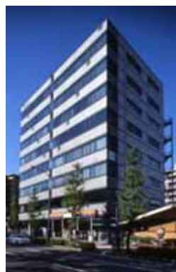
B7 IWATA Building
